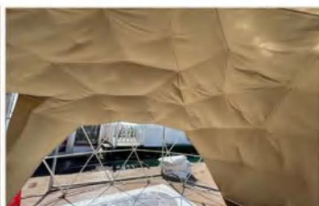
seperated insulation layer canvas layer
