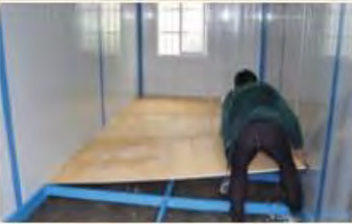
Install The Floor And Roof
